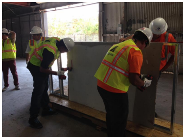
Baker Triangle gives a lesson in installing metal studs and drywall.
